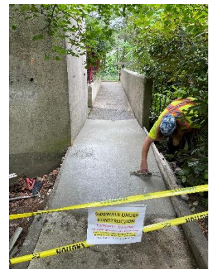
Putting finishing touches on the repaired sidewalk
